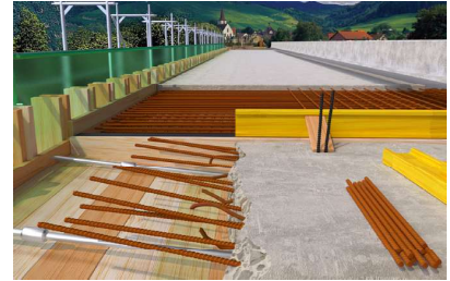
Rebar connections
